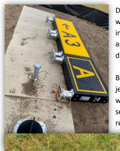
Due to the Earth's composition, magnetic North is constantly moving, which results in magnetic declination (variation). Because runway headings are designated by magnetic headings, runway 4/22 was renumbered and repainted to 5/23. The project replaced infrastructure above and un-
